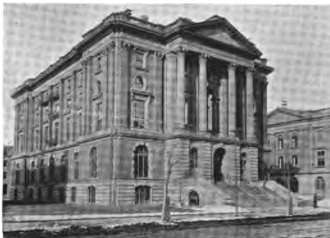
ROGERS BUILDING. MASSACHUSETTS INSTITUTE OF TECHNOLOGY.
